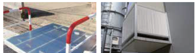
● Installed over the lid of a drainage ditch for water noise control. ● Used in noise control on external ducts
